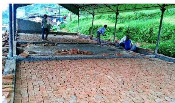
Volunteers laying bricks on top of the concrete
