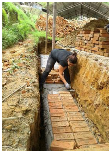
Volunteers laying bricks on dry concrete
