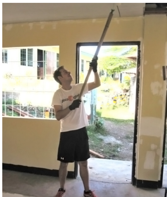
A volunteer works on the ceilings of the classroom.
