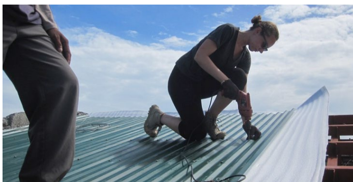
A volunteer working on the roofing.
